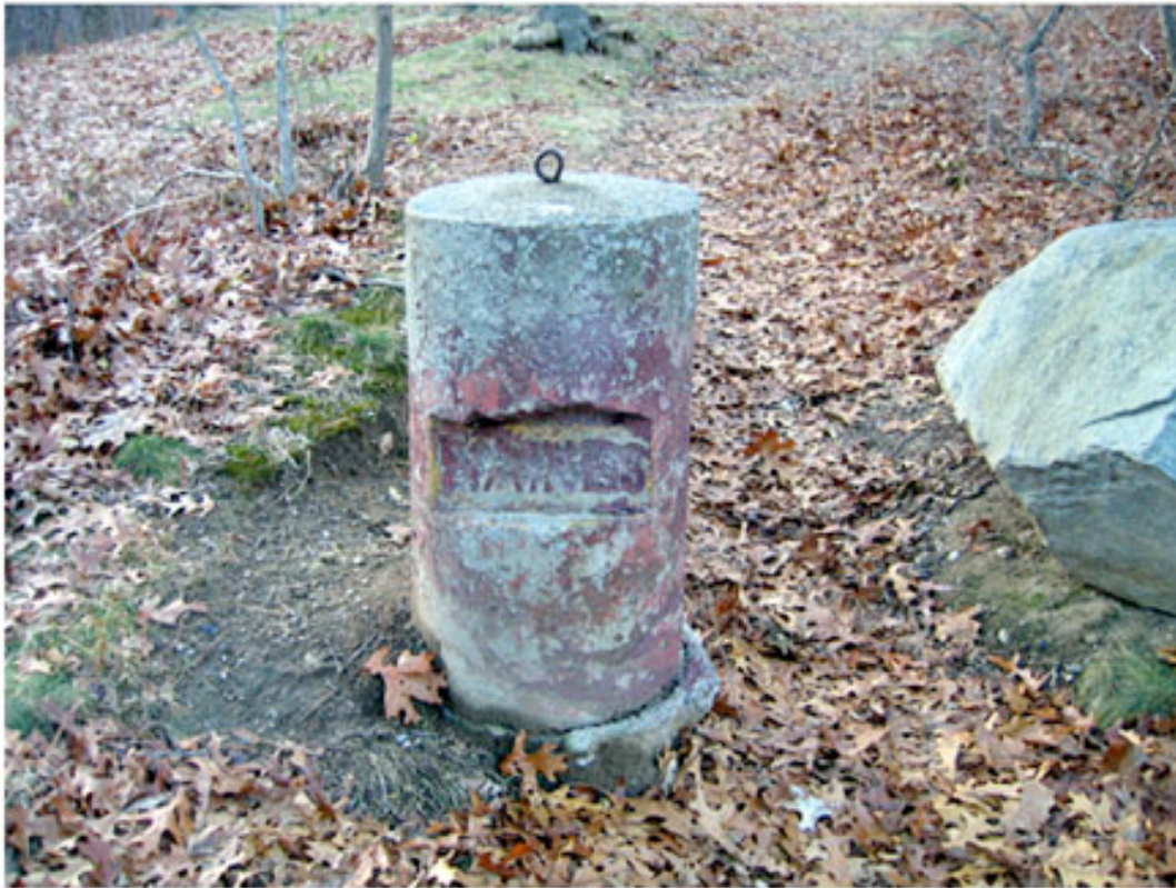
Historic Haines Park marker shows weather damage from 13 years without a coat of paint.
