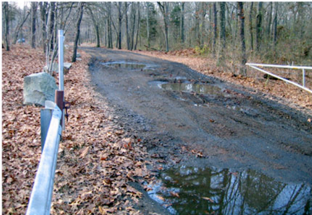
Entrance to west parking lot shows deep potholes in crushed asphalt surface.
